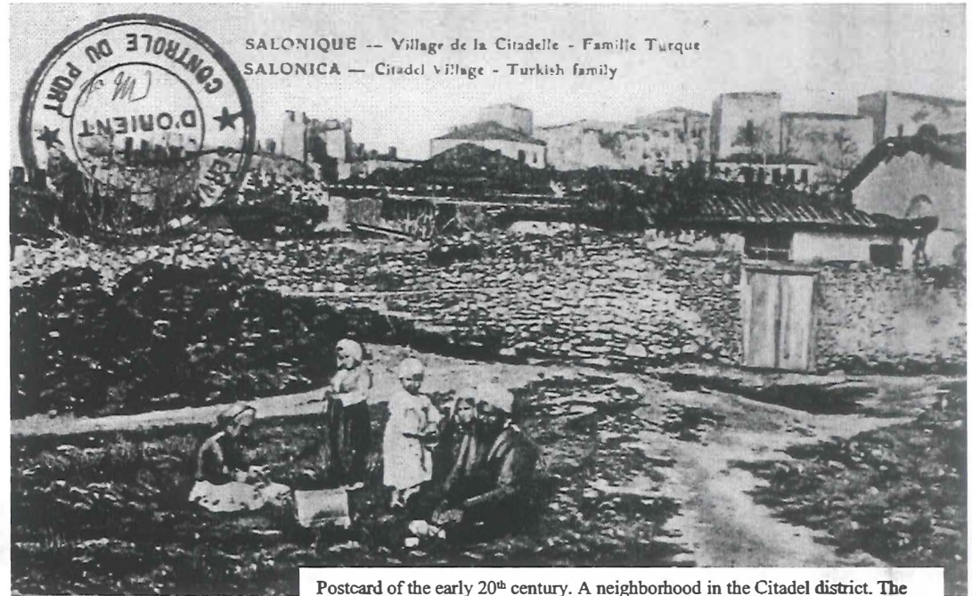
Postcard of the early 20 th century. A neighborhood in the Citadel district. The South side of the Heptapyrgion at the background.
