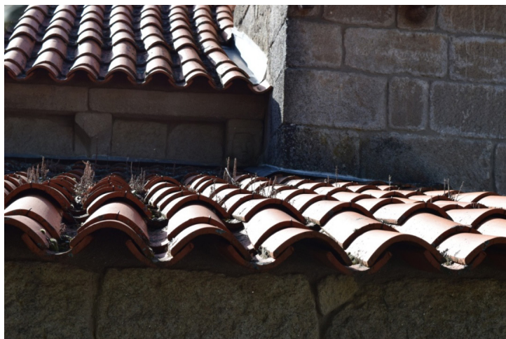
Fig.4. São Tiago Adeganha Church (Torre de Moncorvo, Portugal), HeritageCare inspection 2018-10-22: sacristy roof covering.
