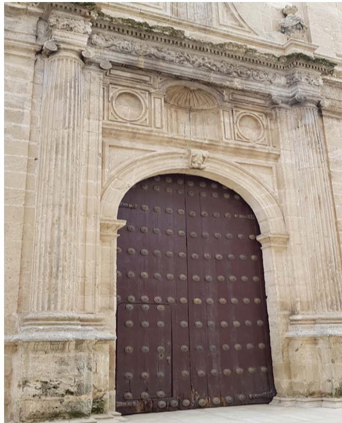
Fig.8. Chapel of the Cinco Llagas Hospital, currently Headquarters of the Regional Parliament of Andalusia (Sevilla, Spain), HeritageCare inspection 2018-10-23: door detail.
