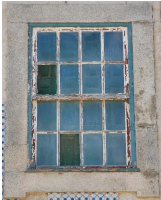
Fig.7. Cantareira Traffic and Telegraphic Station (Porto, Portugal), HeritageCare inspection 20b8-02-20: window frame detail.
