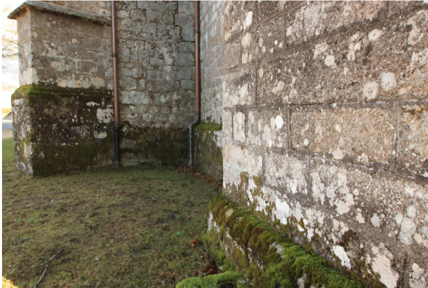
Fig.5. Sainte Croix Church (Rosiers d'Egletons, South West of France), HeritageCare inspection, 2019-02-26.
