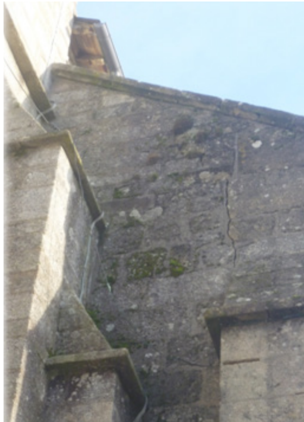
Fig.3. Saint Antoine church (Egletons, South West of France) HeritageCare inspection, 2019-02-27: foundation's settlement linked crack.
