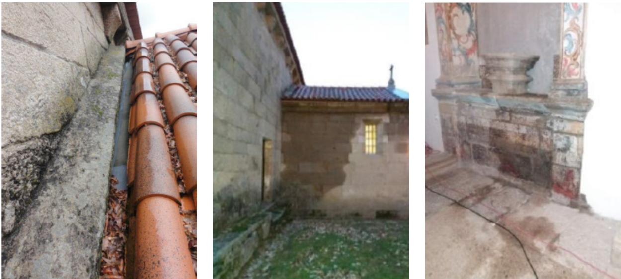
Fig.2. Parish church of Covas do Barroso (Boticas, Portugal), HeritageCare inspection 2018-11-04: water infiltration in the South chapel.
